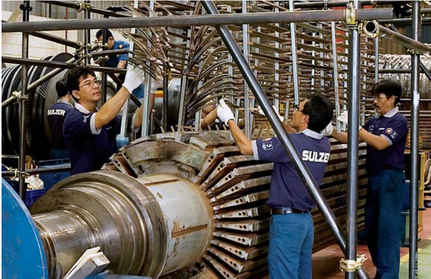
Re-winding works on the generator rotor.
