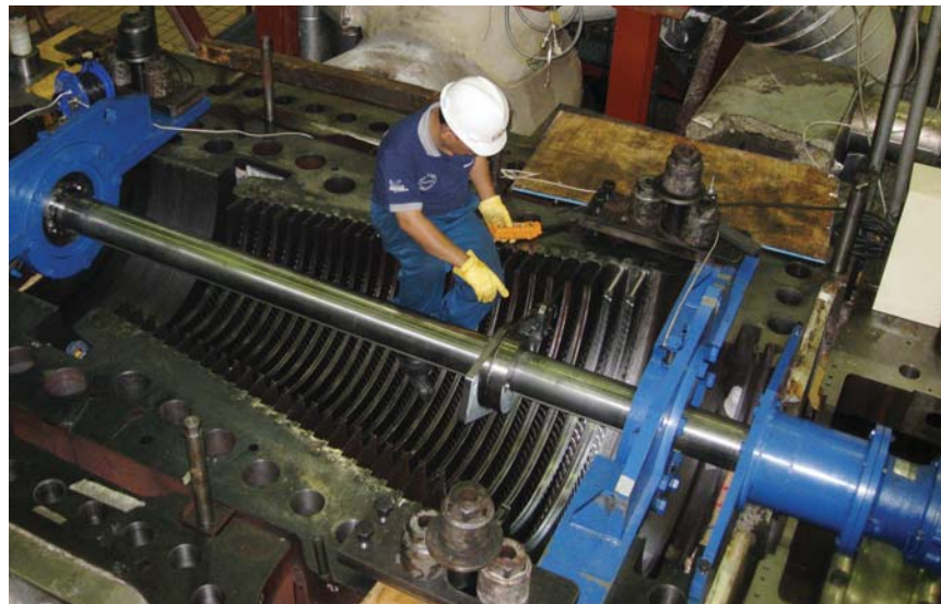
In-situ field machining of HP turbine stationary components.
