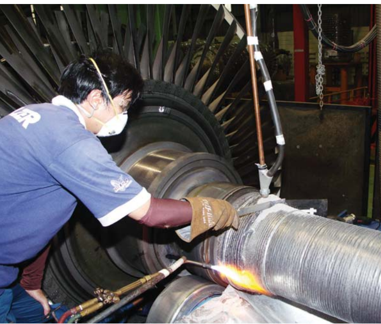
Welding process on the journal of the LP rotor.
