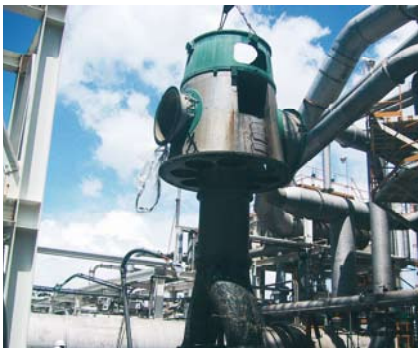
Hot well pump removal for overhaul
