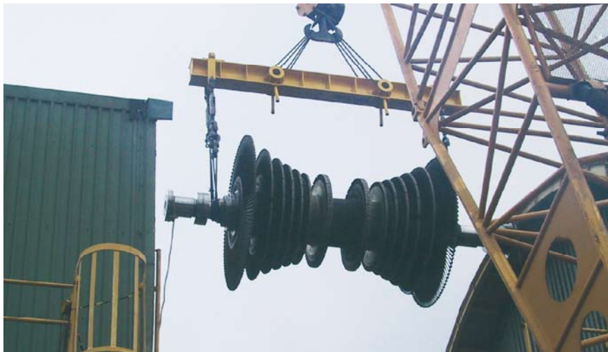
Removing rotor from casing
