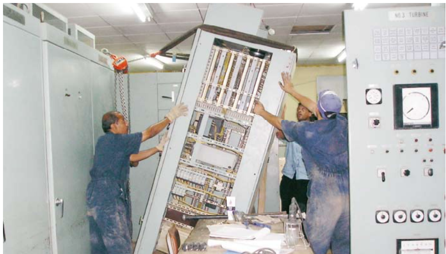
Removing the old turbine controls
