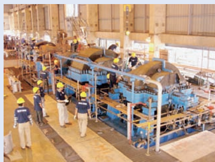
Preparation for upper casing removal.
