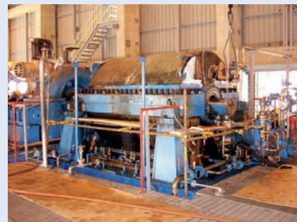
Disassembly of propylene refrigerant compressor.
