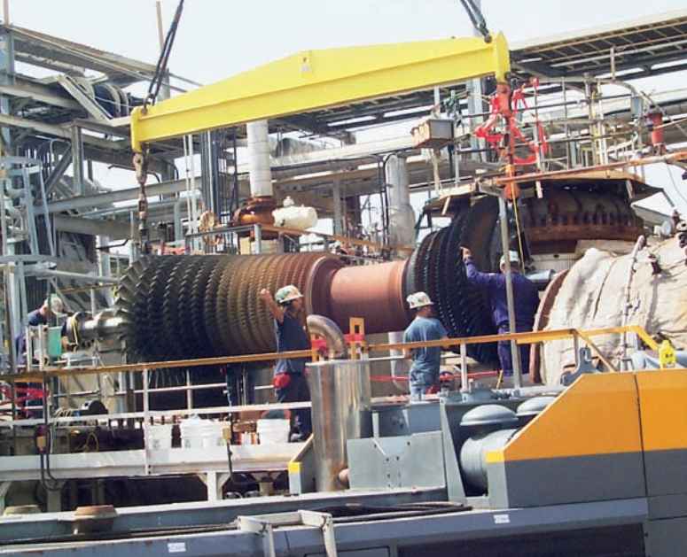
Rotor of MS502 being removed on site.
