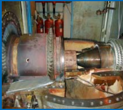
Frame 1 hot gas inspection.
