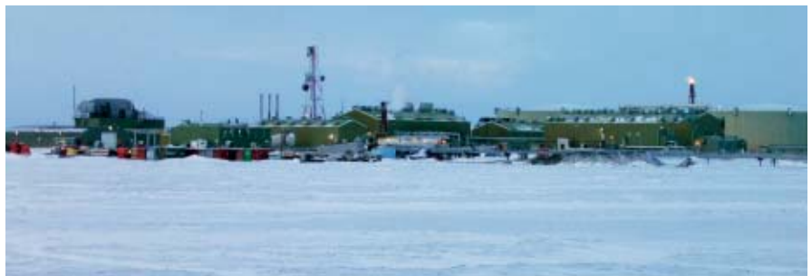
Pump Station 1 North Slope of Alaska.
