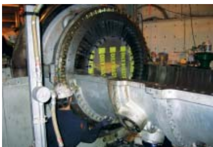
VIGV gear replacement.
