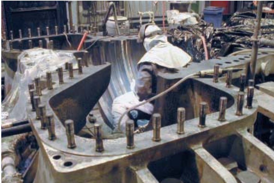
Weld repair to steam turbine in the under casing
