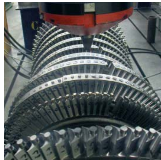
Riveting of a steam turbine rotor
