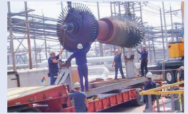
Rotor removal after transportation.
