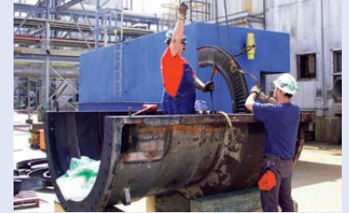
Compressor diaphragm removal.
