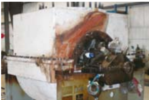
Unit set up for disassembly.
